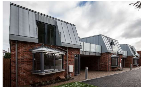
Buckingham Road Housing developed by the Council
