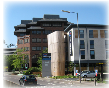
Elstree Way, Borehamwood
