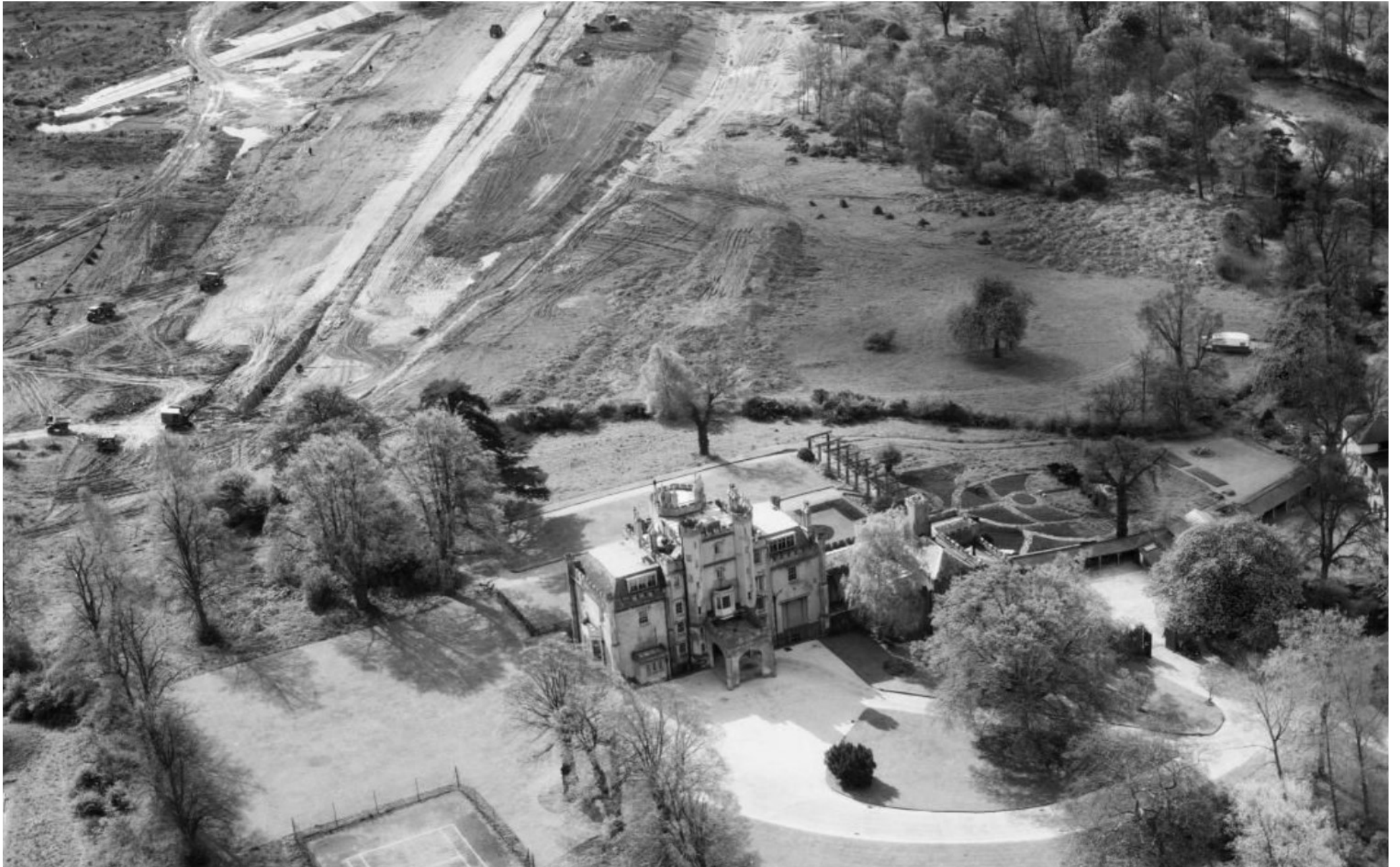
Figure 27: Aerial photograph of the 'Construction of the Hillfield Park Reservoir, Bushey Heath, 1952' (Britain from Above; EAWo48862)
