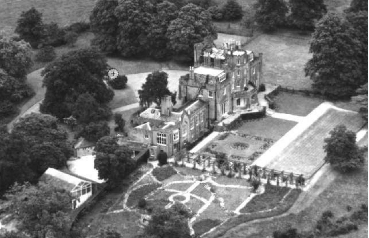
Figure 8 – Detail of Hilfield Castle from the air, as it was in 1949 (Aerofilms EAW 023654). looking at the long south-east elevation.
