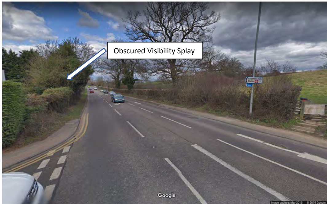
Existing visibility to the left from Carpenders Avenue onto the A4008
