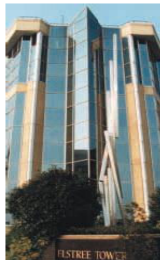
High buildings – emphasising a point of civic or visual significance
