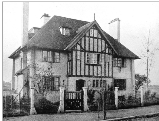
Photograph of Homeleigh , The Avenue (front)
