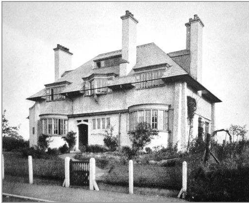
Photograph of Seldown , The Avenue (front)
