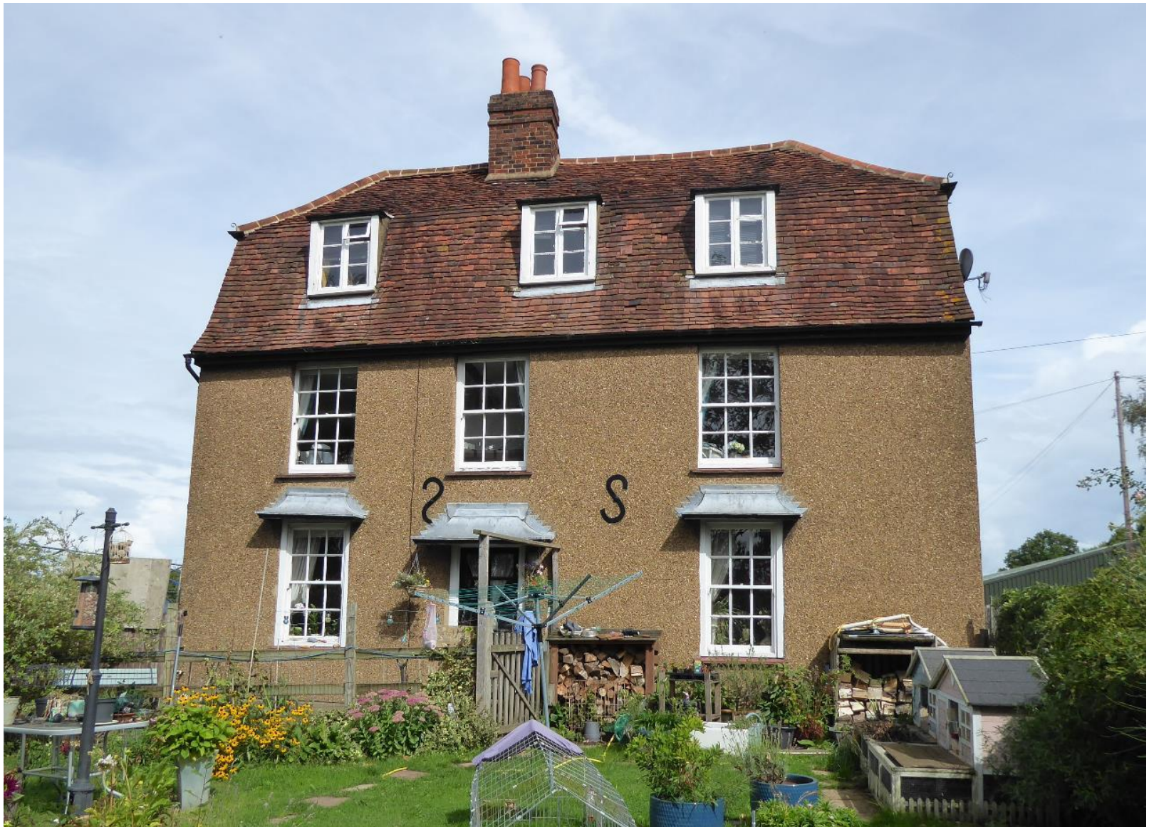
Figure 3: View of Slades Farmhouse from west
