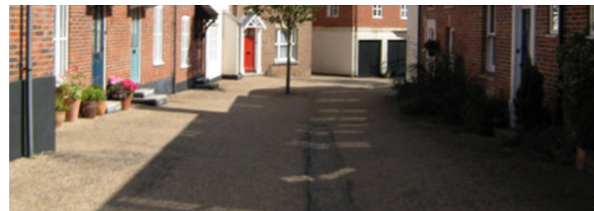
Shared residential Lane, bound gravel on tarmac, not delineation, central drainage
