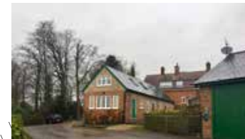
Porters Park Stables Flats & Dairy
