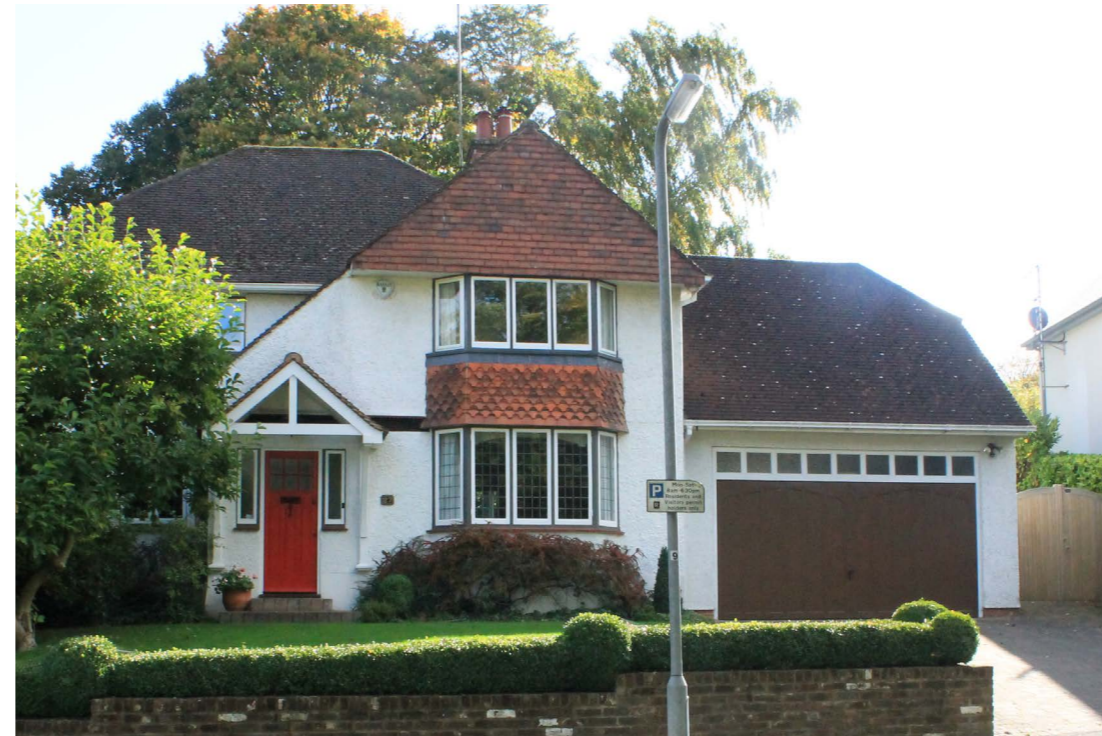
Aldenham Avenue; chalk, render tiles
