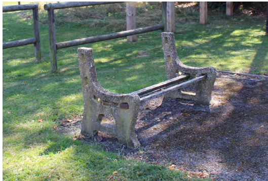
Figure 79 Damaged bench on Blanche Lane
