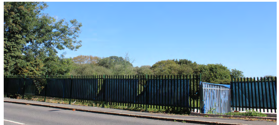
Figure 78 Metal railings on St Albans Road
