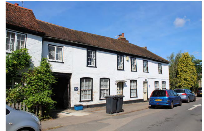
Figure 31 Painted brick elevations of 62 and 64 Blanche Lane
