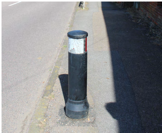
Figure 80 Plastic bollard on Blanche Lane
