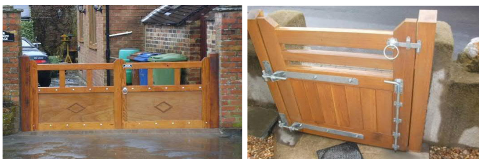
Figure 5-4 Example of flood gates
